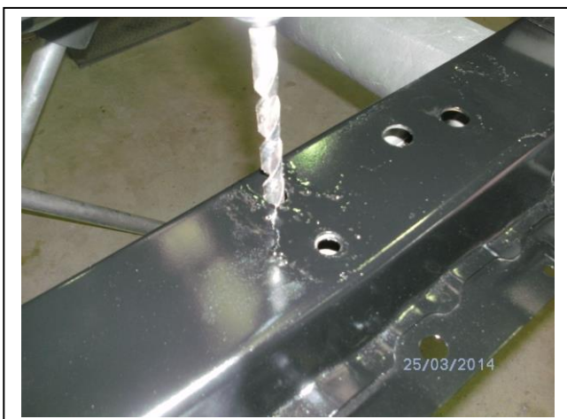
Figure 3: Install ECB tow bracket to drivers side of chassis. Top bolt is accessible when bumper support removed.
